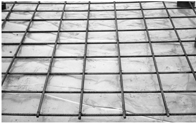
Fig. 1.7—Reinforcing bar in concrete slabs placed directly on vapor retarder help to control slab curling and cracking. Supported deformed bars no smaller than No. 4 (No. 13) should be used, and the bars spaced far enough apart so workers can step between them (Holland and Walker 1998).
