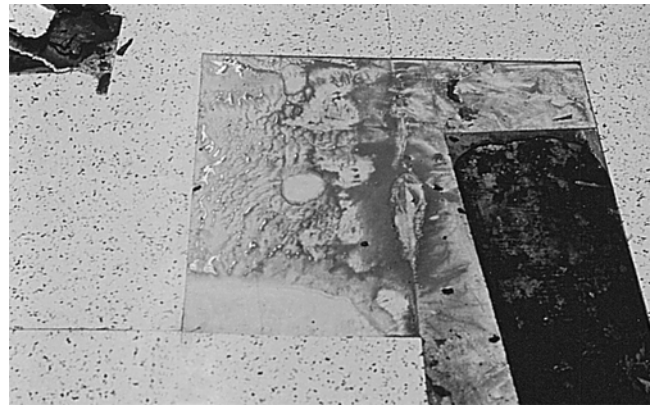
Fig. 1.4—Adhesive degradation leading to debanded solid vinyl tile installed over asbestos tile. (Courtesy of Peter Craig.)
